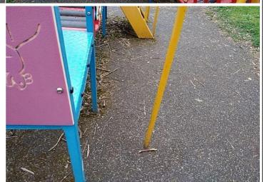
**Finding:** The firemans pole is less than 350mm from the platform and does not meet with the recommendations of BS EN 1176 Part 1
